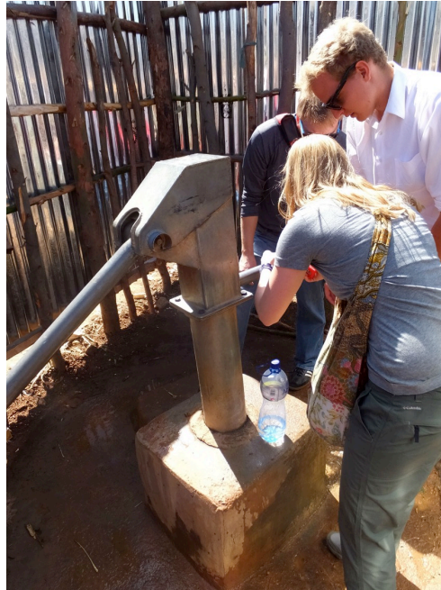
Well # 2 30 m, almost dry
