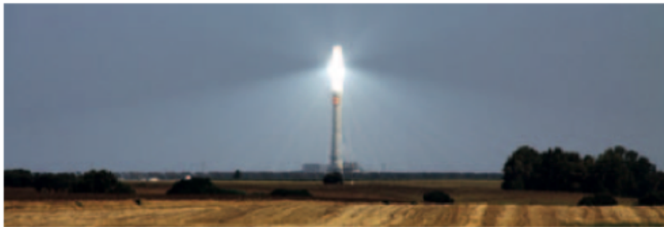
Photo 3.1 The Gemasolar power tower near Sevilla (Spain)
