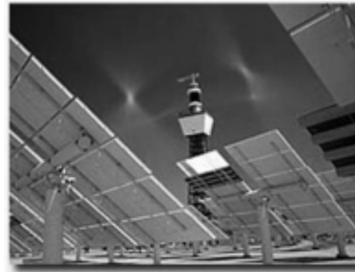
FIGURE 10.7 Heliostat detail of the Solar Two plant (source: www.energy.lanl.gov/sunlab/overview.htm ).
