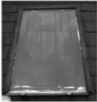
Figure 4-7 A home-made clip fin collector.
