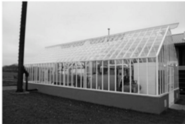
Fig. 5. Biochar plant in Denmark, with 35 KWe cogeneration capacity, powered by Stirling engine.
