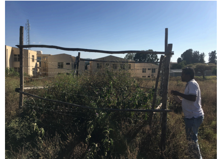
Well and Solar Pump
