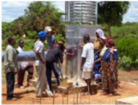
Figure 2. Local people helped install the solar icemakers.
